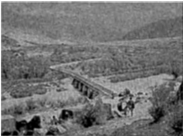
FIG. 5. Inverted siphon and mouth of tunnel 'Kazerun'.
